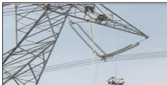
Fig. 8: Robot installation using rope
