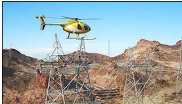
Fig. 6: Helicopter inspection of PL
