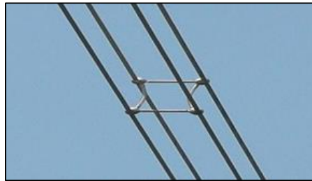
Fig. 10: Bundled conductors
