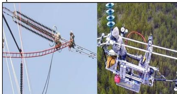
Fig. 5: Service personnel working on energized lines
