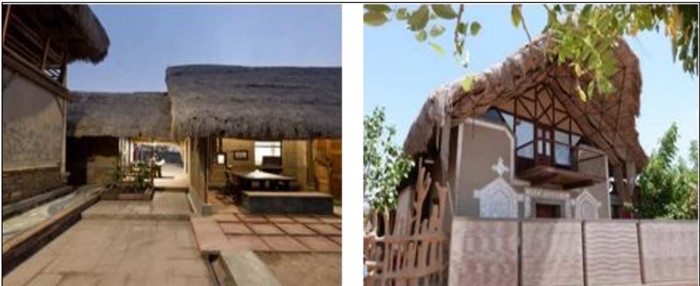
Fig. 2: Prototype structures on campus made with traditional building techniques
