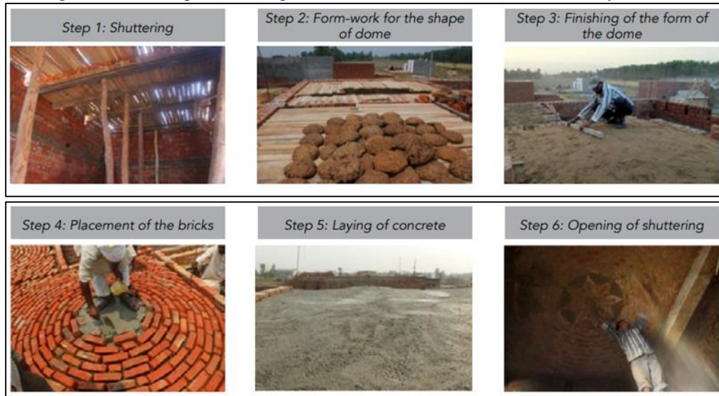
Fig. 8: Stepwise construction of the dome
