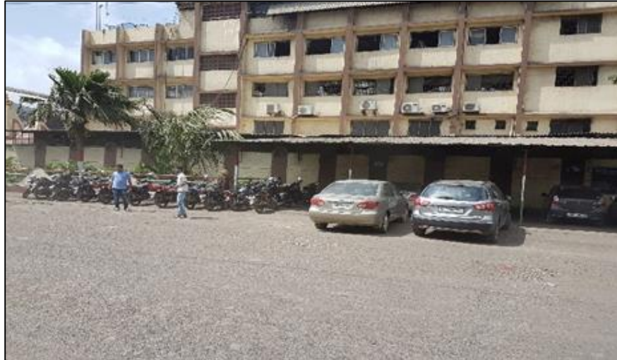
Fig. 12: Existing Parking Condition
