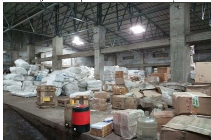
Fig. 8: Existing warehouse condition
