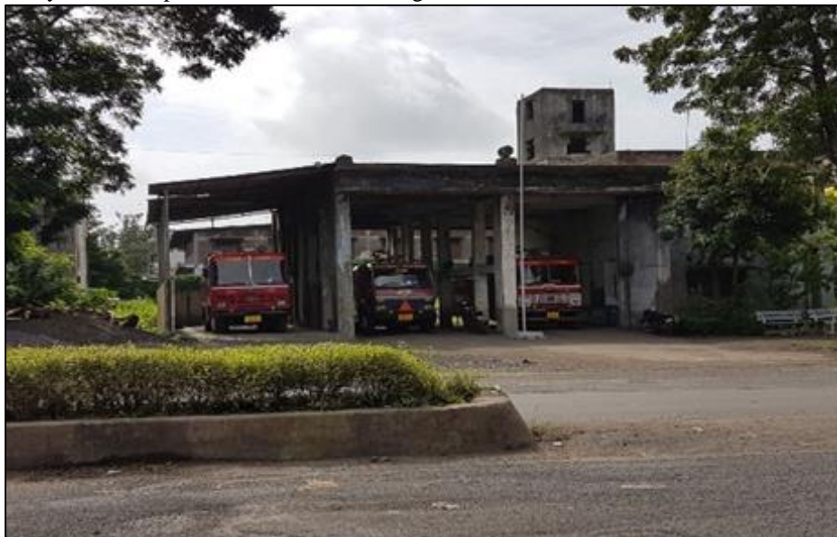
Fig. 6: Existing fire station condition
