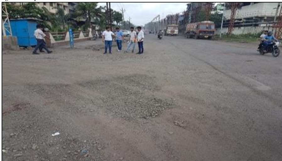
Fig. 5: Existing Roadway Condition at Sachin G.I.D.C
